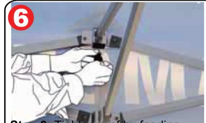
**Step 6:** Tighten roof by feeding straps around the lower truss bars. Once clipped in, pull down on the strap until firm.
